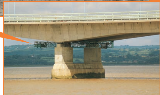
Access Gantry on Second Severn Bridge
