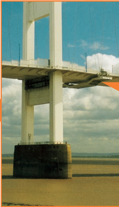
Access Gantry on Severn Bridge
